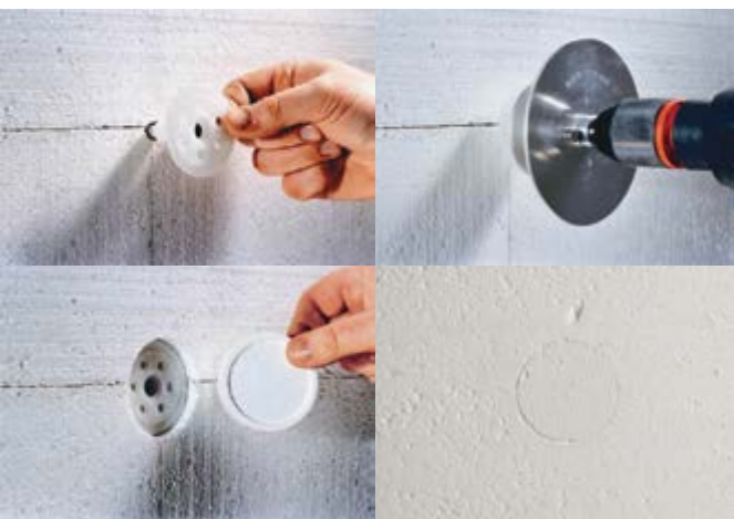
StoTherm Anchor installed on timber frame.
