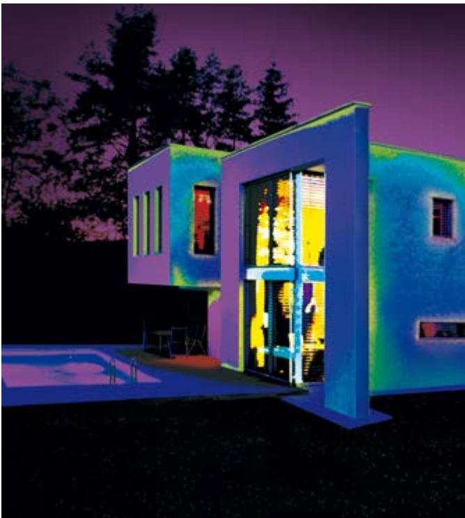
StoTherm insulation through thermography.
