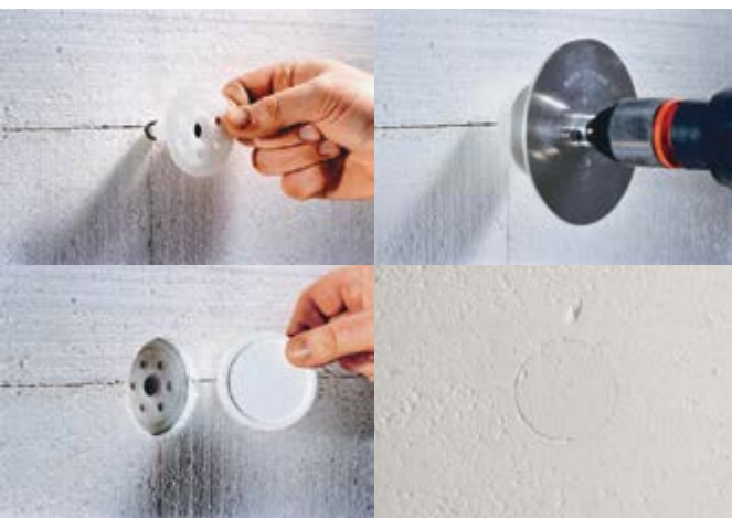
StoTherm Anchor installed on timber frame.
