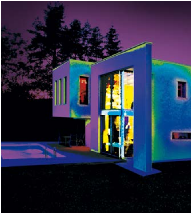
StoTherm insulation through thermography.
