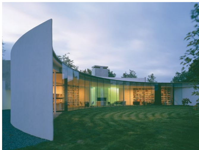
Above: Residential house, The Crescent in Wiltshire, Great Britain Architect: Ken Shuttleworth, Sir Norman Foster
