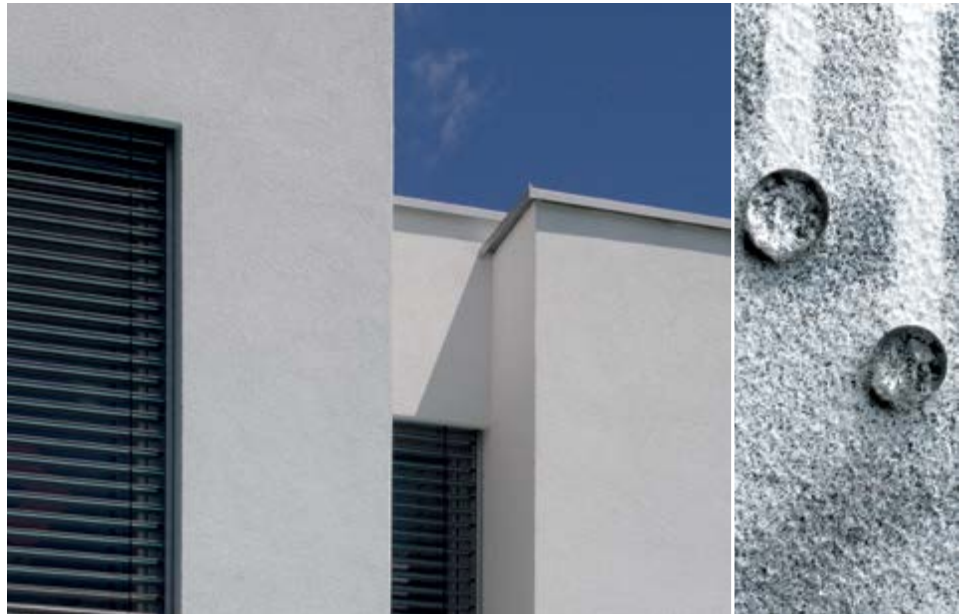
The problem with conventional facades is that soiling becomes more and more visible over time. Above all, dirt deposits and moisture on the structurally unprotected weather sides provide an ideal breeding ground for micro-organisms.
