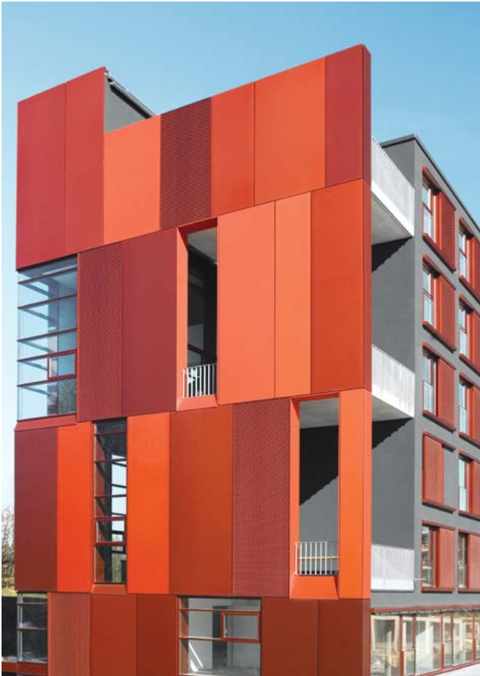
Student Housing, München, Germany Architectural firm: Spengler + Wischolek, Hamburg, Germany
