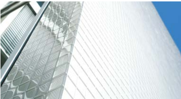
StoVentec M with glass mosaics Gewoge Haus, Brunnckstr, Ludwigshafen Architectural firm: Allmann Sattler Wappner, München, Germany
