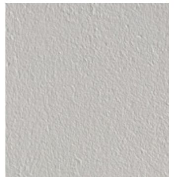
StoMiral Render: Bagged mineral render, coated with StoColor facade paint.
